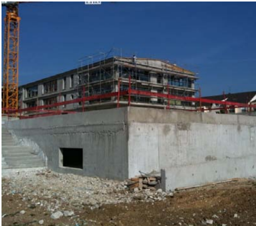
The east wing end of September 2009
