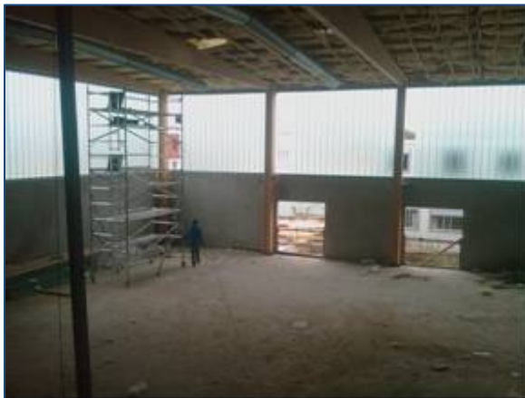
The completed roof on the multi-purpose hall
