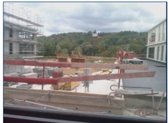
Terrace under construction
