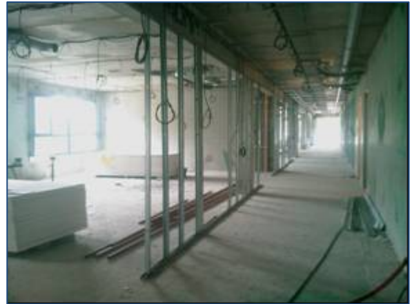
The classroom partitioning being erected
