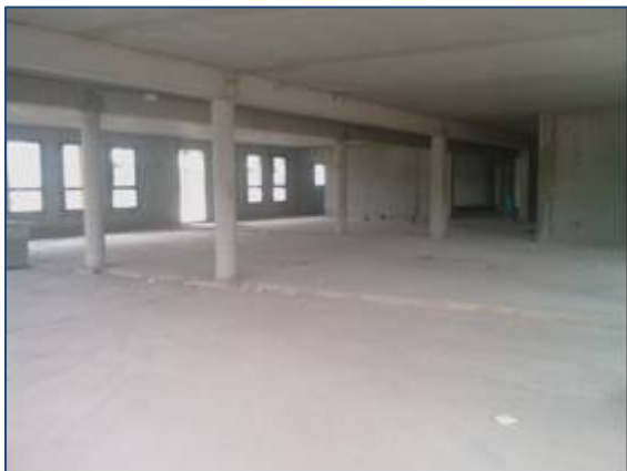
The school refectory
