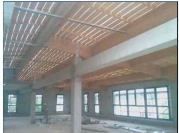
The roof under construction and window installation
